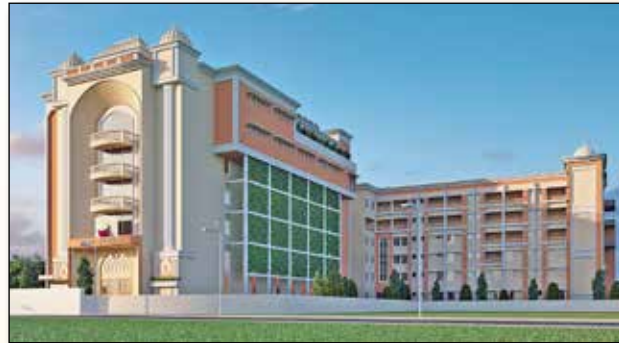
Artist's rendering of Advaita Ashrama's new publications building currently under construction in Kolkata, India.
