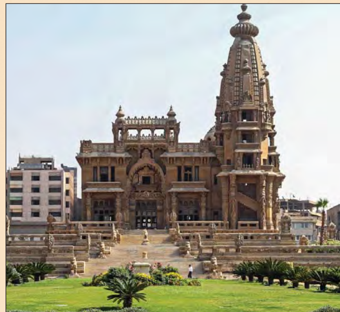
The Hindu Palace: The structure was designed by the French architect Alexandre Marcel (who also created the cinema La Pagode in Paris) and built following the then-revolutionary process of reinforced concrete. Of Khmer inspiration, it is impressive for its rich ornamentation, with images of snakes, Buddhas and Hindu Shivas, Krishnas and other Deities. The garden is a botanical paradise of marvels, now restored, that the baron gathered during his travels.
