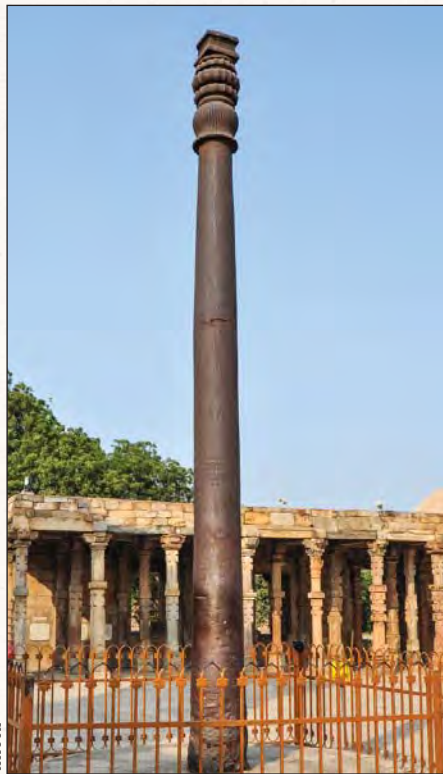
Magical Gupta metallurgy: Originally established in Madhya Pradesh in 402 ce by Chandra Gupta II in honor of Vishnu, the famed iron pillar was moved to Qutab Minar, Delhi, by Sultan Iltutmish. Mysteriously, it has remained free of corrosion for over sixteen centuries.
